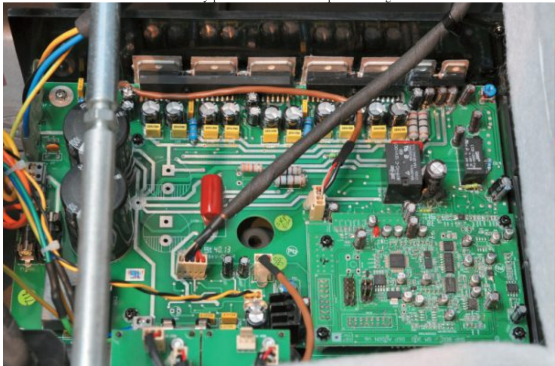
The electronics inside, equipped with five power amplifiers ICs and the DSP board placed at the lower right
